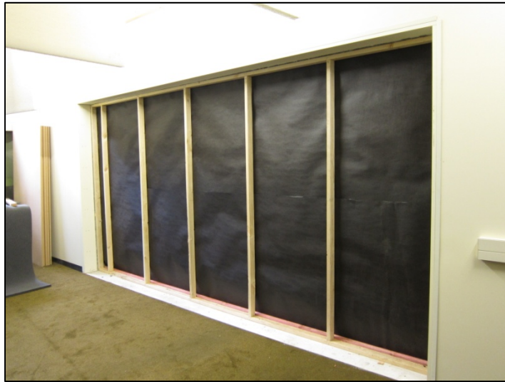
Figure 12: Underlay as viewed from the semi-anechoic room side.
