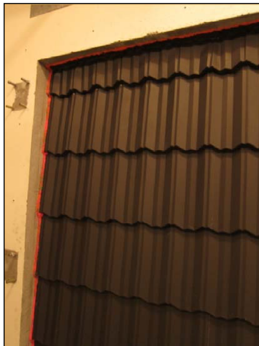
Figure 5: Metal tiles with the top row of tiles bent at the top of the concrete opening.
