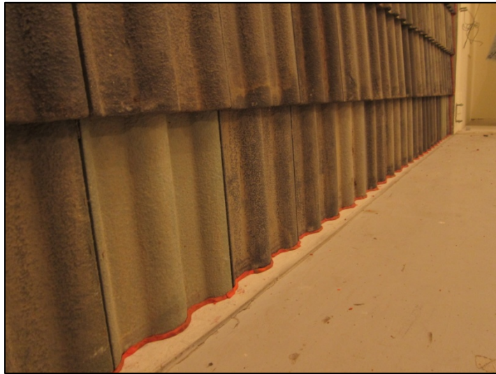
Figure 10: Bottom row of the concrete tiles showing the sealing compound.
