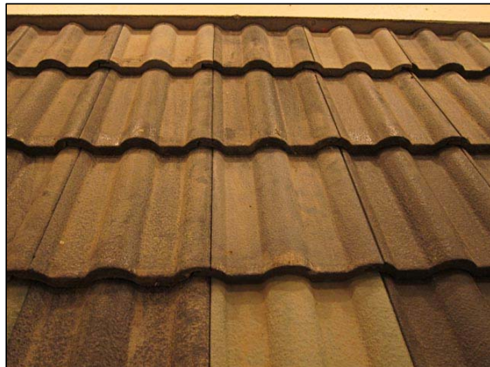
Figure 9: Concrete tiles nailed to battens as viewed from the reverberation room side of the test opening.
