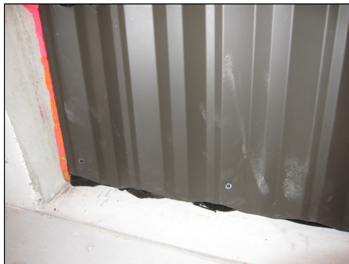
Figure 7: Resilient material located between the bottom row of tiles and the concrete floor.
