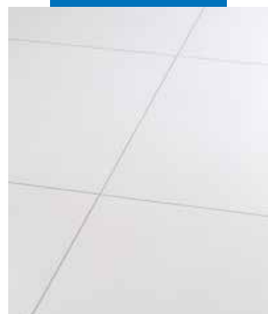
Flooring grouted with Ultracolor Plus
