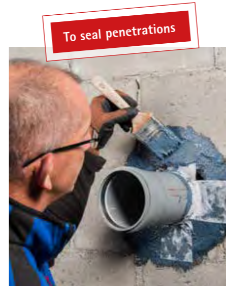
To seal detail features with lots of edges and corners
