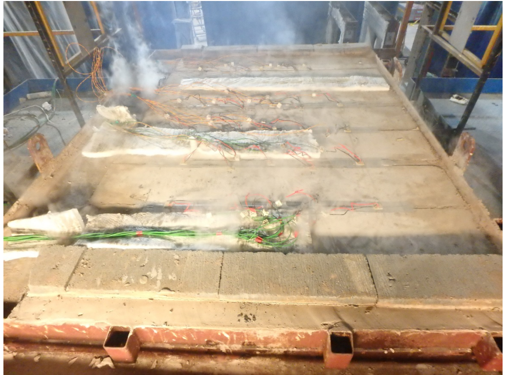
The unexposed face of the floor assembly after a test duration of 120 minutes
