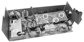
**Step 4:** Remove all 5 connections to the circuit board as highlighted below.
