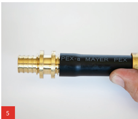
Ensure fitting is inserted
