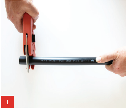
Cut pipe at right angle
