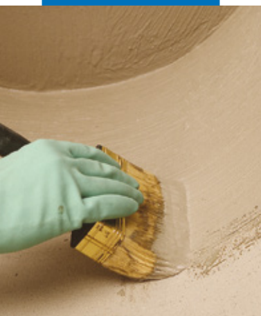
Waterproofing of details by brush
