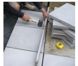
STEP 9. Check levels across pavers continuously and tap down if needed.
