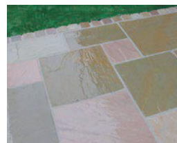
STEP 12. Sweep off the remainder of the grout 45 degree to the grout lines.
