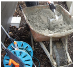
STEP 5. Mix PREMIER-MORTAR-MIX with water to toothpaste consistency (in a wheelbarrow or mixer) or mix PREMIER-WASHED-SAND with cement, water and plasticiser - sand and cement can be ordered from Premier Group.
