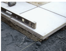
STEP 10. You should end up with approx 40mm paver, 20mm mortar, 60mm base. When all pavers are laid - DO NOT WALK ON FOR 24 HOURS.
