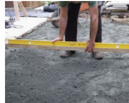
STEP 4. Check levels with spirit level.
