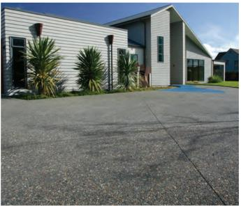
While we have taken care to give an accurate representation of our READY Exposed range, aggregates are natural products, so some variations in colour and stone size will occur. Placing, weather and site conditions may also influence the end result. The examples shown have been sealed.
