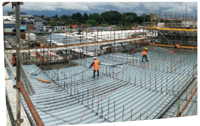
Mason Apartments – Otahuhu, Auckland using Tray-dec 80
